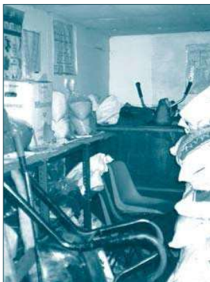
An untidy trading hut presents hazards to users
